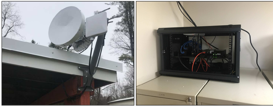
RSA/MDS installed a B Site antenna and cabinet housing the modem, router, and necessary wiring to extend Wi-Fi service at a VFW Hall in Linesville, PA.
