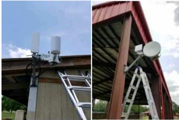
RSA/MDS installed A Site and B Site Antennas in Castle Hayne, NC.
