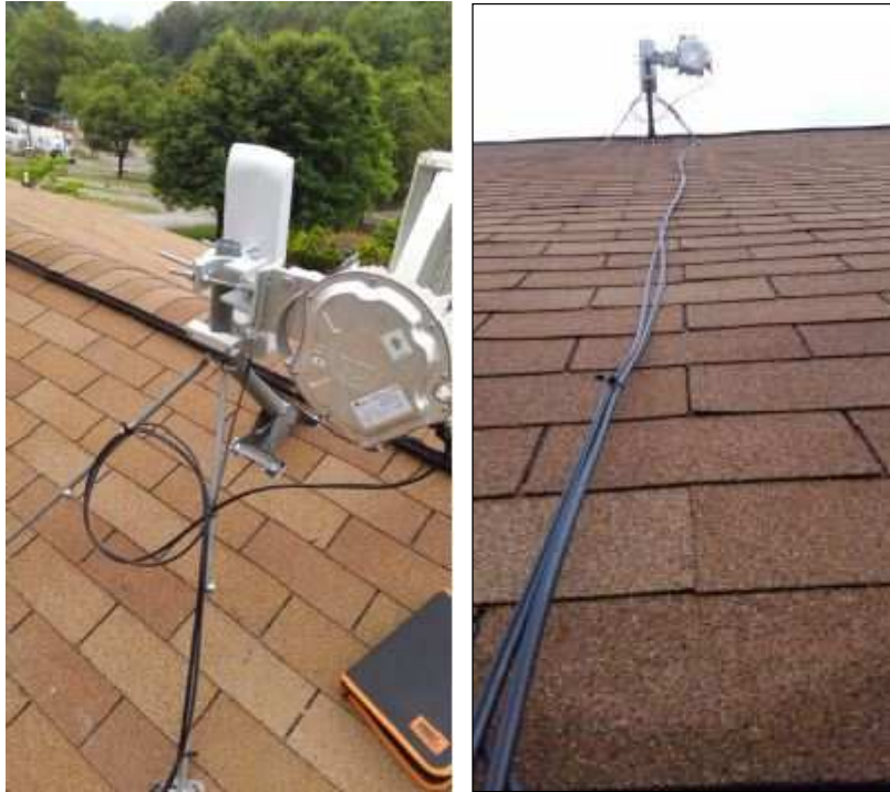
RSA/MDS mounted an A Site Antenna and CAT5 Routing Cable to the roof of a building at a KOA campsite in Blountville, TN.
