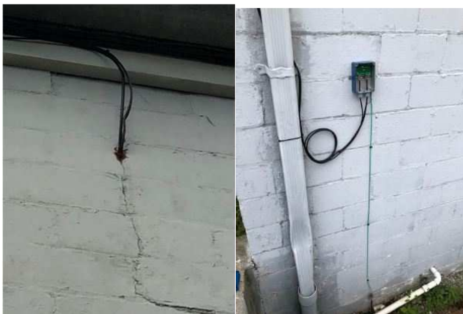
Installations often require wall penetration, weather-proofing, and lightning protection/grounding, including this installation at a Fanelli Boys location in Parkersburg, WV.
